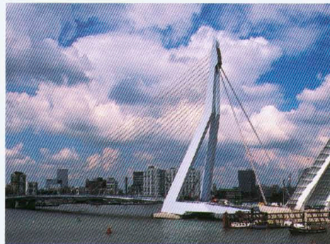
Erasmus Bridge, Rotterdam, The Netherlands, 1990-1996
